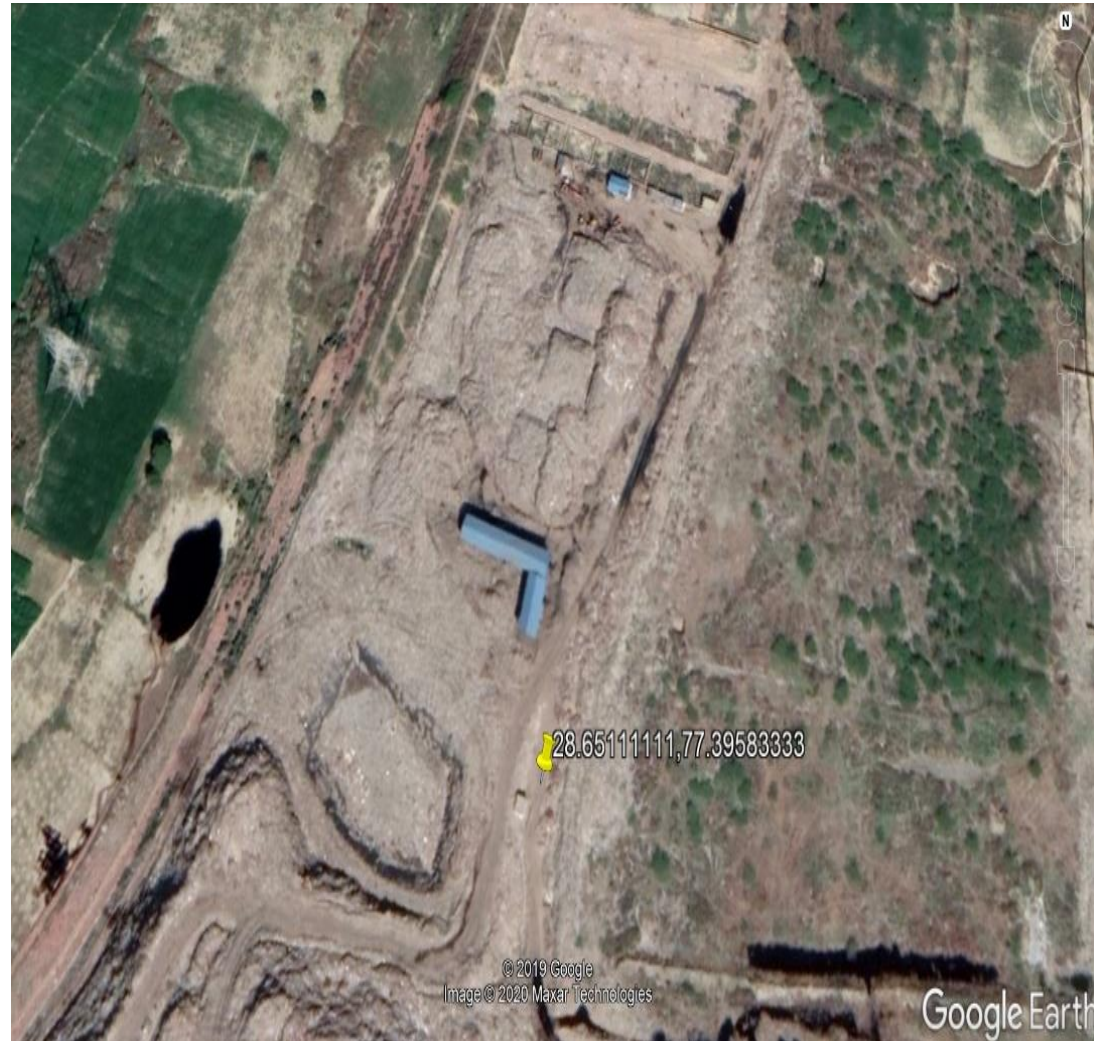
Figure 16: Satellite image of Pratap Vihar Solid Waste Management Plant
